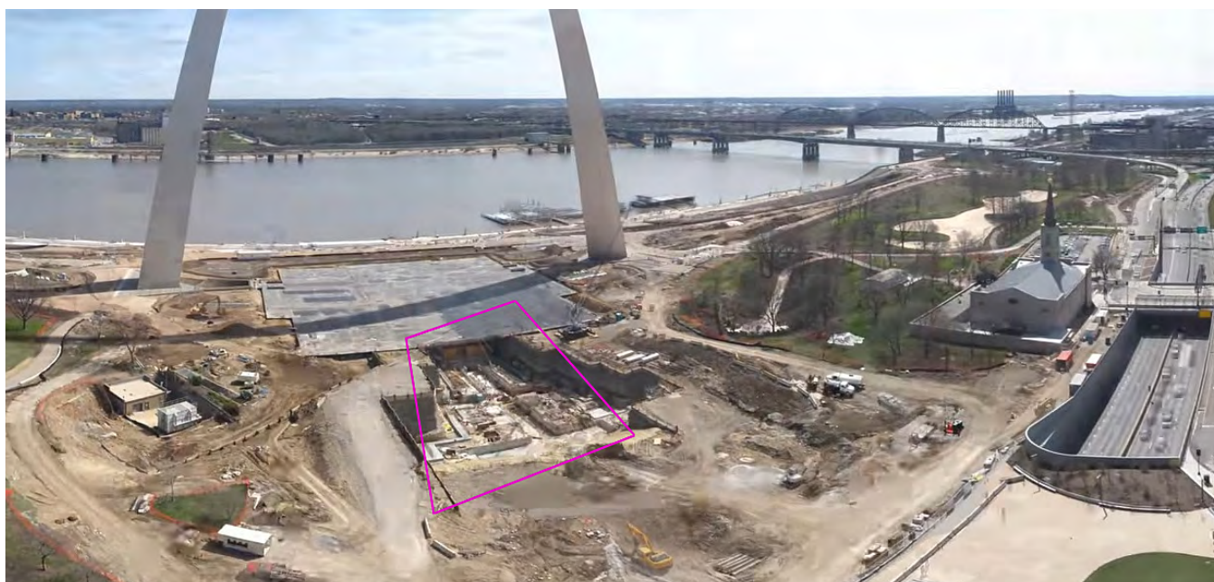
Fig. 3 - Under construction – a 46,000 square-foot expansion to the Gateway Arch Park includes a new visitors center and museum expansion. At this point in the construction, utility tunnels (indicated by shaded area above) were built below publicly accessible areas to provide a pathway for utility lines and to allow workers to move about without entering public areas. The interior of these cast-in-place, below grade concrete tunnels were later treated with Xypex Crystalline Waterproofing Technology. (Photo courtesy of EarthCam)
