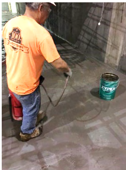
Fig. 5 & 6 - The St. Louis branch of Western Specialty Contractors (WSC) applied (see first photo) a slurry of Xypex Concentrate and Modified crystalline waterproofing to nearly 20,000 square feet of concrete utility tunnels, drains, and knee walls as part of the expansion and restoration of the Gateway Arch National Park. Workers used handheld sprayers to keep the Xypex coating moist to aid the curing process. (see 2nd photo)
